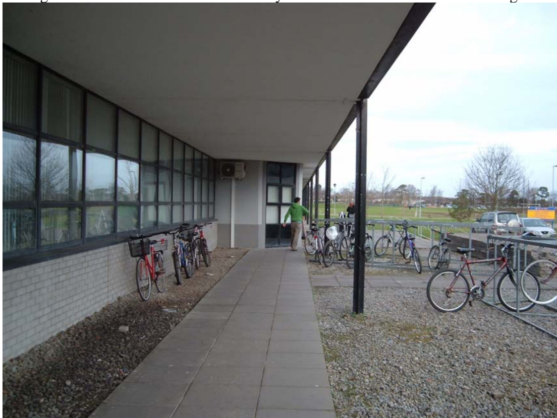
Figure 2: Suitable area for covered bicycle rack installation at Arts Building
